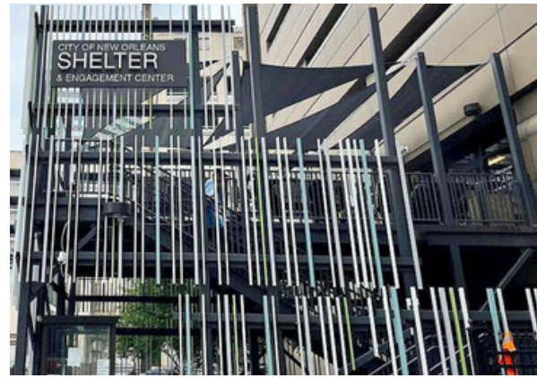
City of NOLA Low Barrier Shelter 40,000SF Renovation Cost $4,180,750 Interior built out to increase the current shelter's capacity by 200%.
