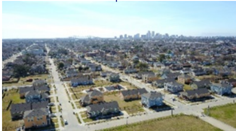
HANO, Florida and Guste Developments Cost $8,288,132 Correction and completion of 156 residential units.
