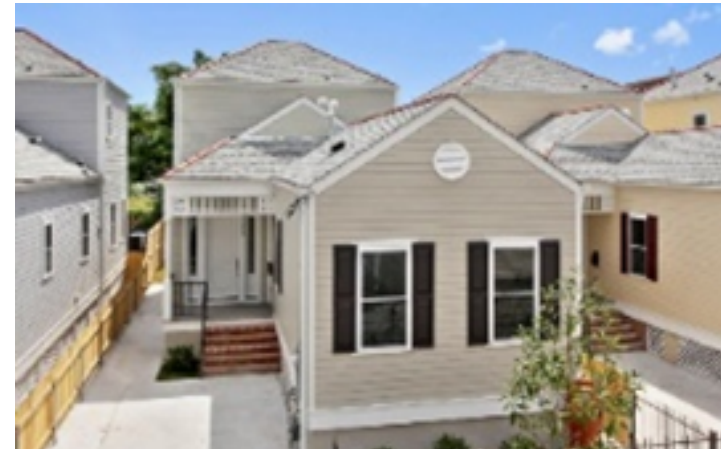
NORA; Saratoga Development Cost $1,546,363 2000SF Constructions of Energy Star and Green Communities.
