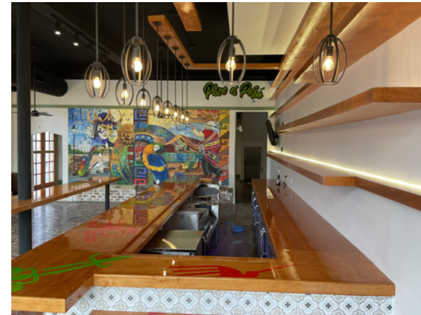
Tito's Ceviche Cost $718,812 Restaurant total renovation of 4582 SF.
